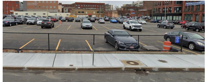
The design and appearance of the Buffum Street Lot is generally unwelcoming.
